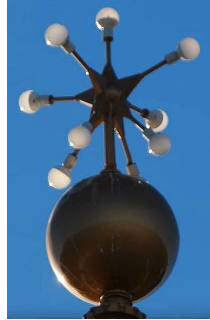
Refurbished Temple Finial
