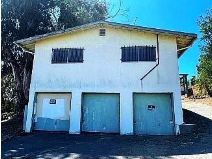
No. 5 Canyon Drive house from below, showing two levels, the lower of which accommodates a three-car garage.
