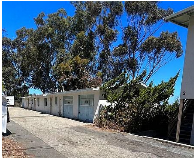
Three-Plex and Two Garages, looking west
